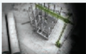
Design, Engineering & Consulting
